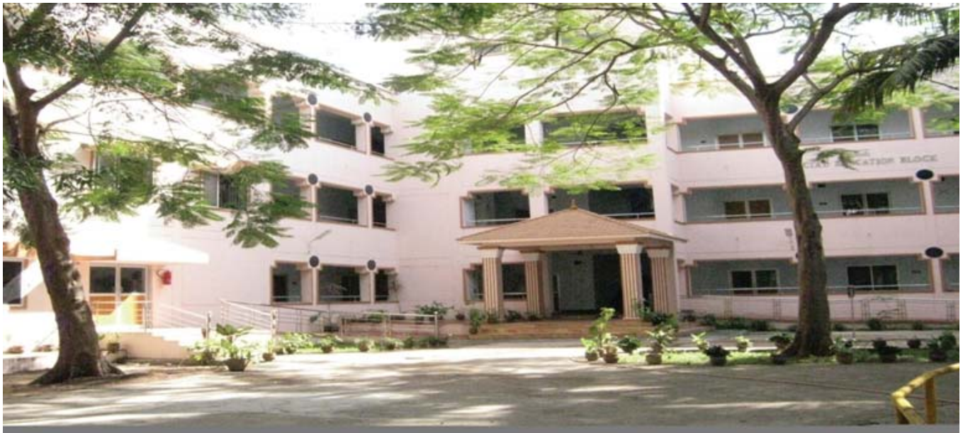
Newly constructed building for running B.Ed. Special Education (Visual Impairment) course at Regional Centre, Chennai
